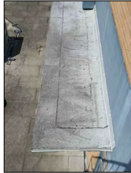
PHOTO # 16 ROOF AREA E4
