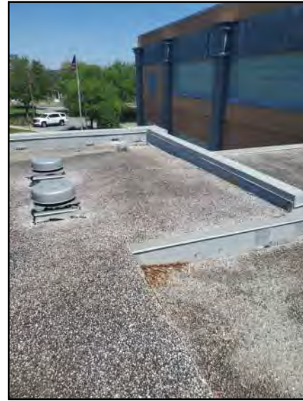
PHOTO # 2 ROOF AREA D
