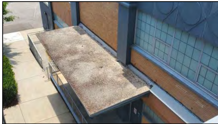
PHOTO # 23 ROOF AREA H
