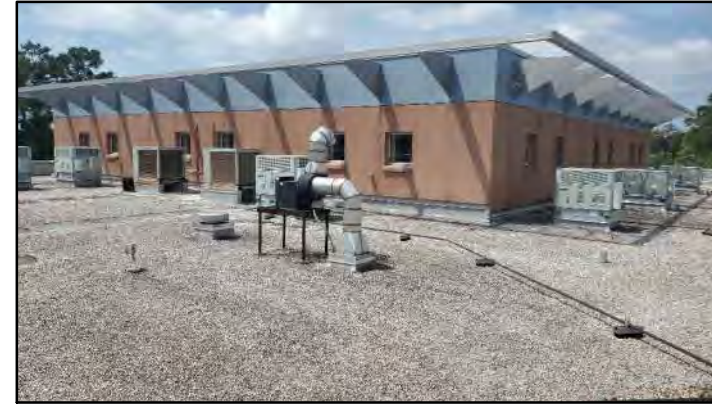
PHOTO # 3 ROOF AREA B
