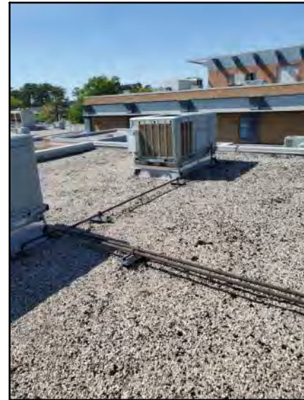
PHOTO # 20 ROOF AREA F
