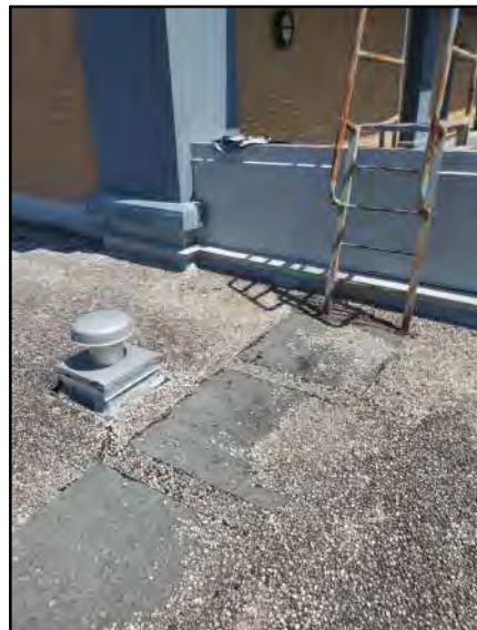
PHOTO # 9 ROOF AREA D1
