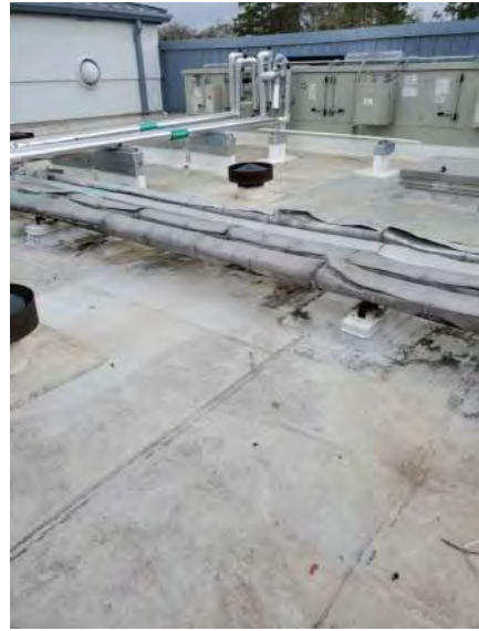
PHOTO # 1 ROOF AREA F
