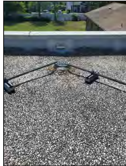
PHOTO # 6 ROOF AREA D
