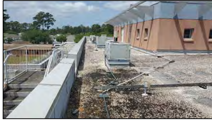
PHOTO # 1 ROOF AREA B
