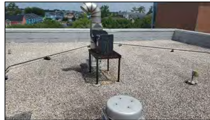
PHOTO # 9 ROOF AREA B
