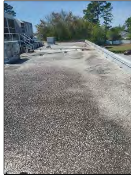
PHOTO # 3 ROOF AREA D
