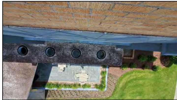
PHOTO # 22 ROOF AREA G
