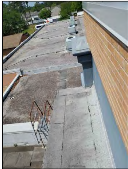
PHOTO # 18 ROOF AREA E4
