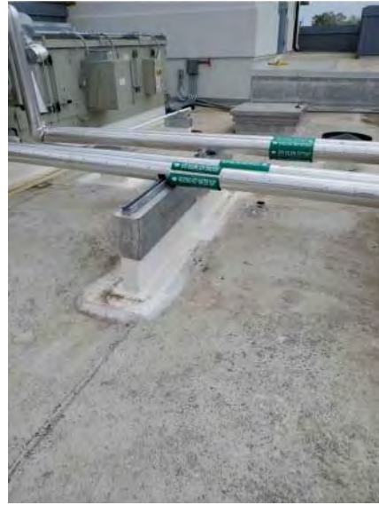
PHOTO # 7 ROOF AREA F
