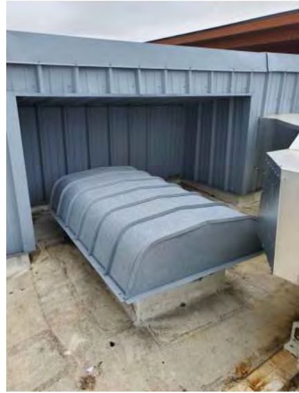
PHOTO # 5 ROOF AREA F
