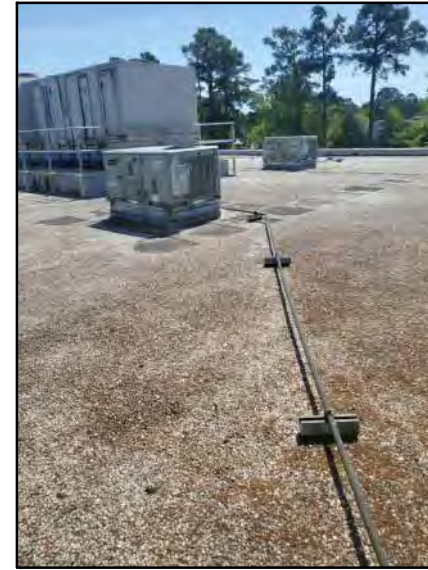
PHOTO # 4 ROOF AREA D
