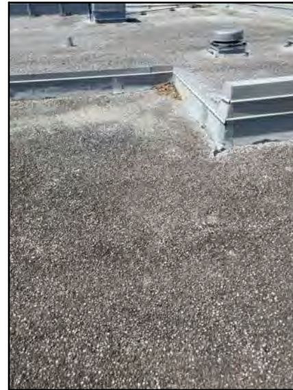
PHOTO # 7 ROOF AREA D1
