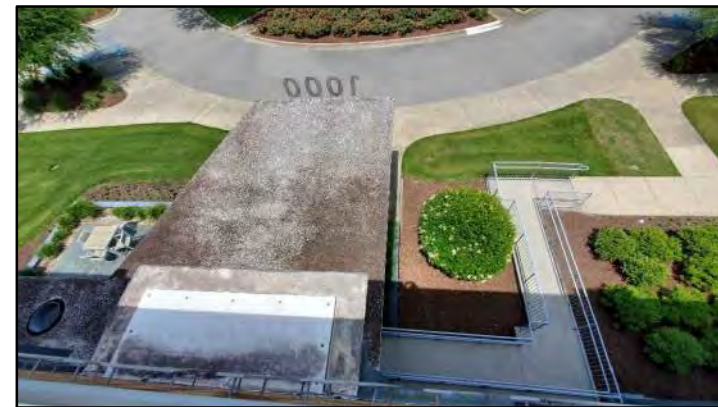
PHOTO # 21 ROOF AREA G
