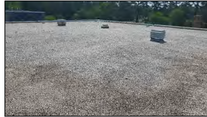
PHOTO # 18 ROOF AREA C
