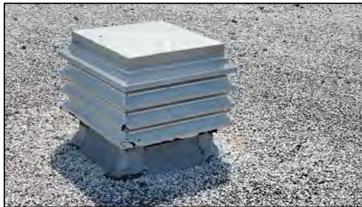
PHOTO # 20 ROOF AREA C
