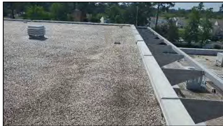
PHOTO # 19 ROOF AREA C
