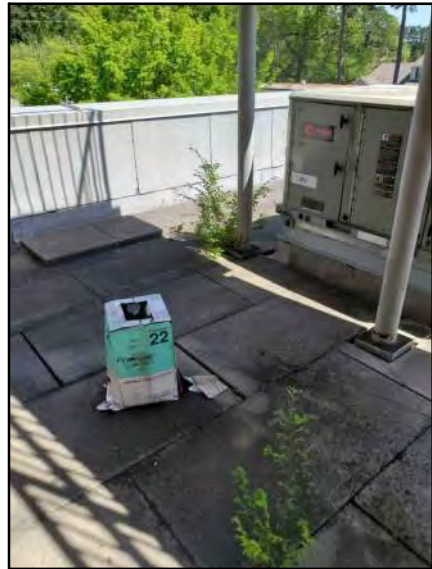
PHOTO # 6 ROOF AREA E
