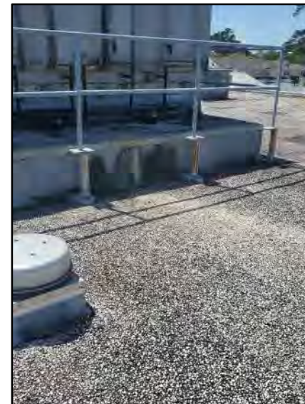
PHOTO # 12 ROOF AREA D2
