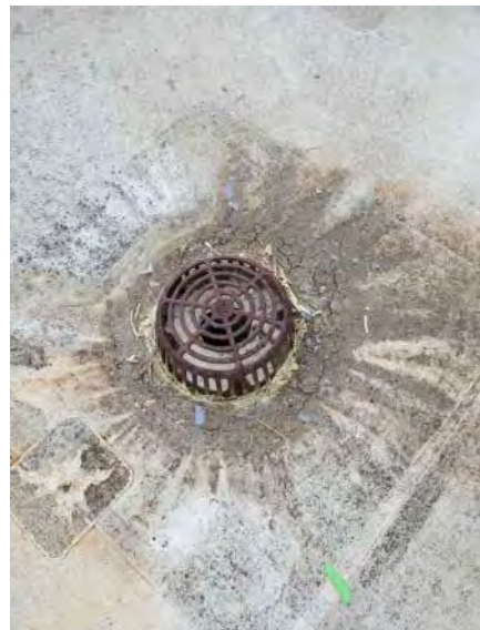
PHOTO # 9 ROOF AREA F
