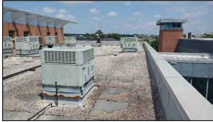
PHOTO # 2 ROOF AREA B
