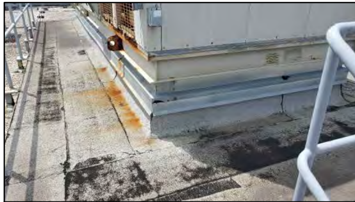
PHOTO # 11 ROOF AREA B1
