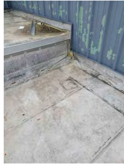
PHOTO # 4 ROOF AREA F
