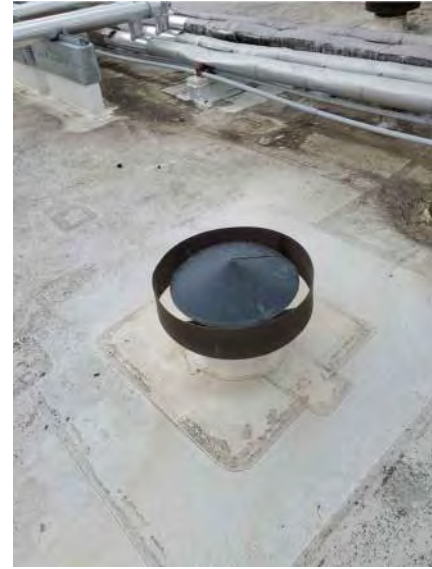
PHOTO # 8 ROOF AREA F
