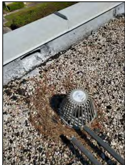
PHOTO # 21 ROOF AREA F
