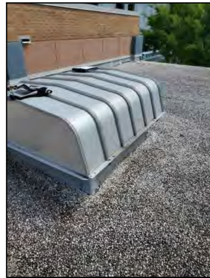
PHOTO # 12 ROOF AREA E2
