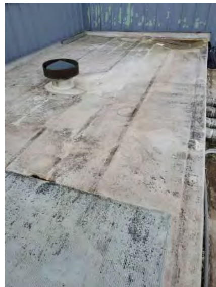
PHOTO # 11 ROOF AREA G
