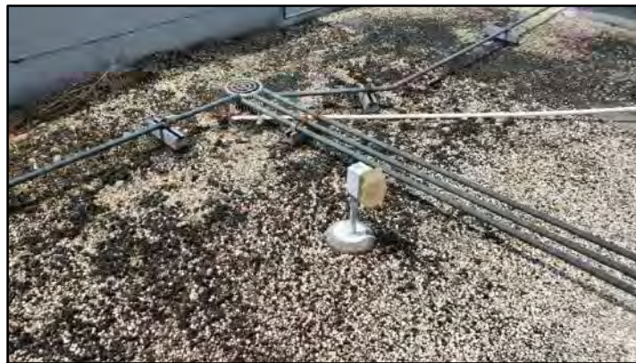
PHOTO # 8 ROOF AREA B
