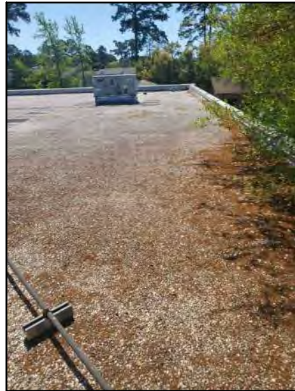
PHOTO # 5 ROOF AREA D
