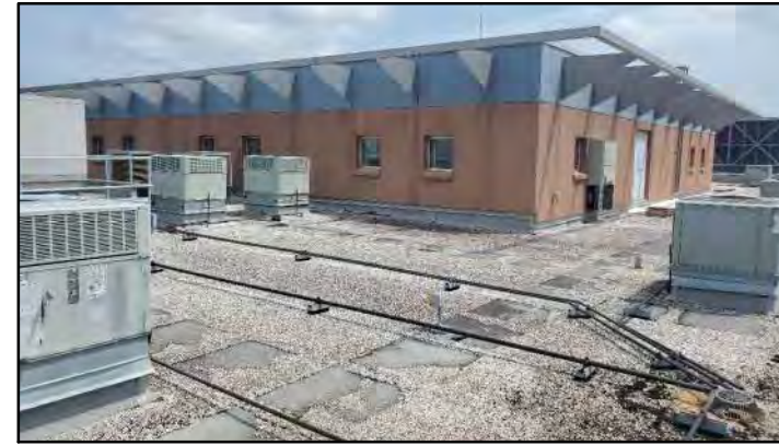
PHOTO # 6 ROOF AREA B
