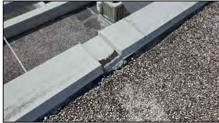
PHOTO # 16 ROOF AREA C
