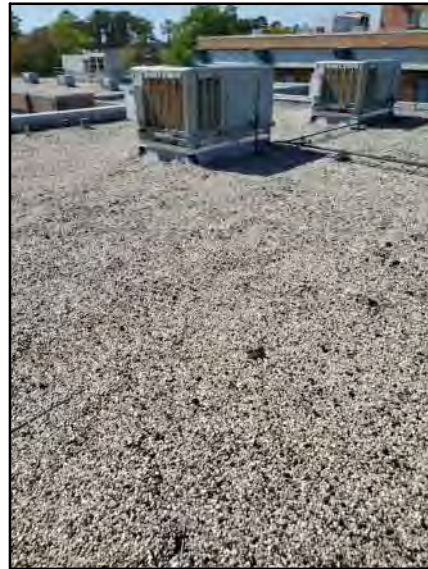
PHOTO # 19 ROOF AREA F
