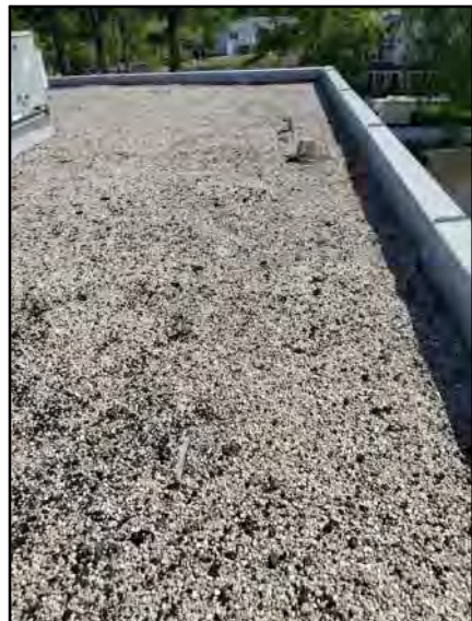
PHOTO # 22 ROOF AREA F
