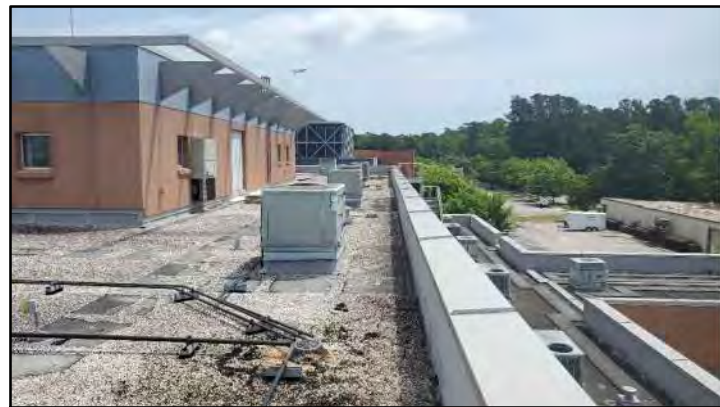
PHOTO # 7 ROOF AREA B
