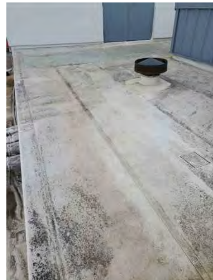
PHOTO # 12 ROOF AREA G
