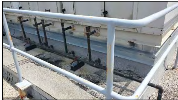
PHOTO # 10 ROOF AREA B1
