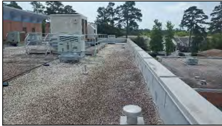
PHOTO # 5 ROOF AREA B
