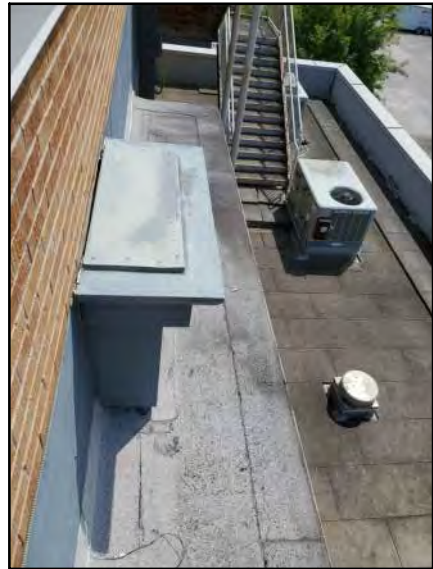
PHOTO # 17 ROOF AREA E4
