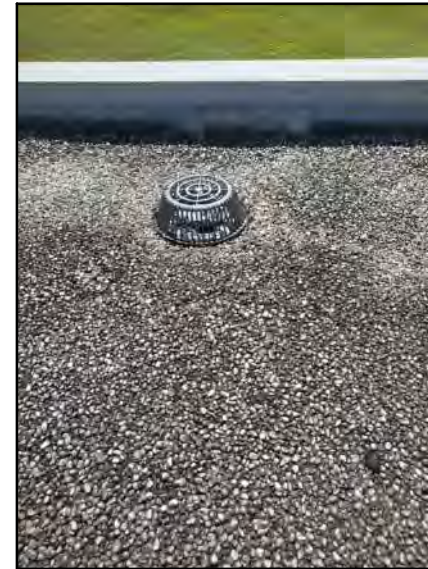
PHOTO # 8 ROOF AREA D1
