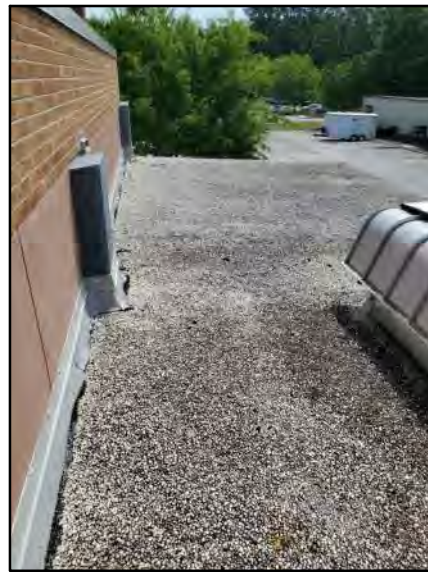
PHOTO # 11 ROOF AREA E2
