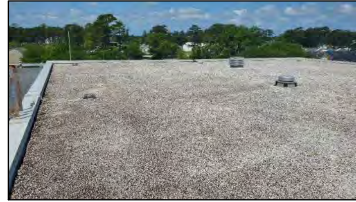
PHOTO # 15 ROOF AREA C
