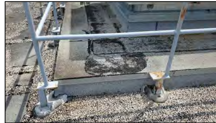
PHOTO # 12 ROOF AREA B1
