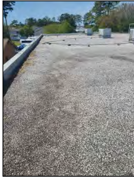
PHOTO # 1 ROOF AREA D
