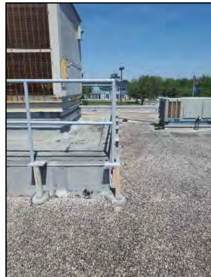
PHOTO # 10 ROOF AREA D2
