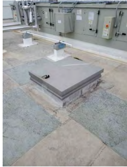
PHOTO # 6 ROOF AREA F
