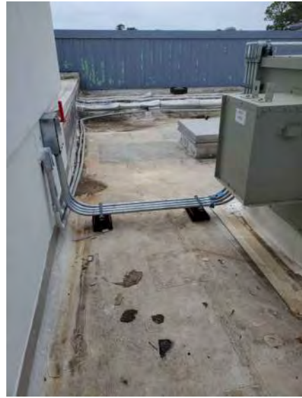
PHOTO # 2 ROOF AREA F
