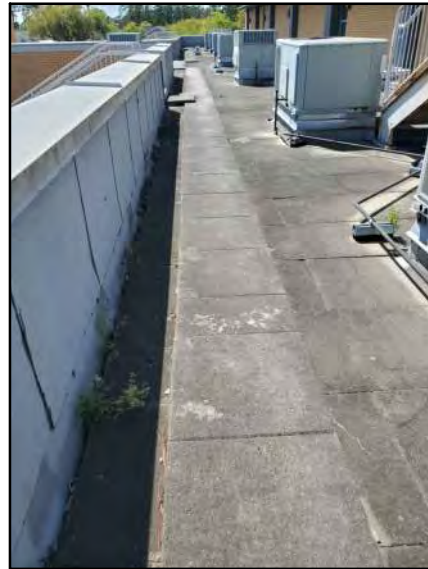
PHOTO # 7 ROOF AREA E
