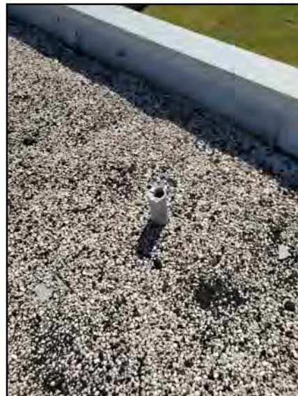
PHOTO # 23 ROOF AREA F
