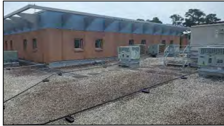
PHOTO # 4 ROOF AREA B
