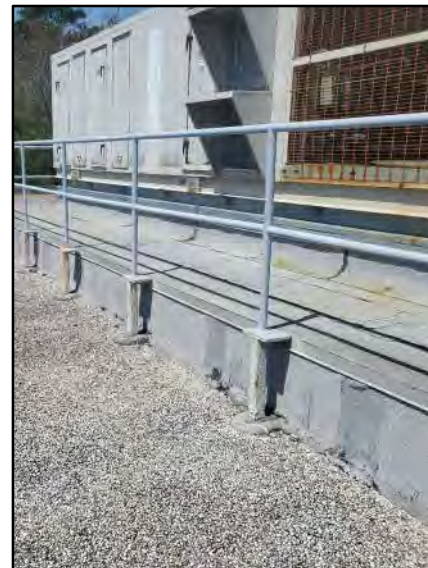
PHOTO # 11 ROOF AREA D2
