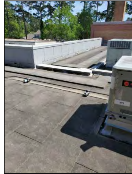
PHOTO # 4 ROOF AREA E
