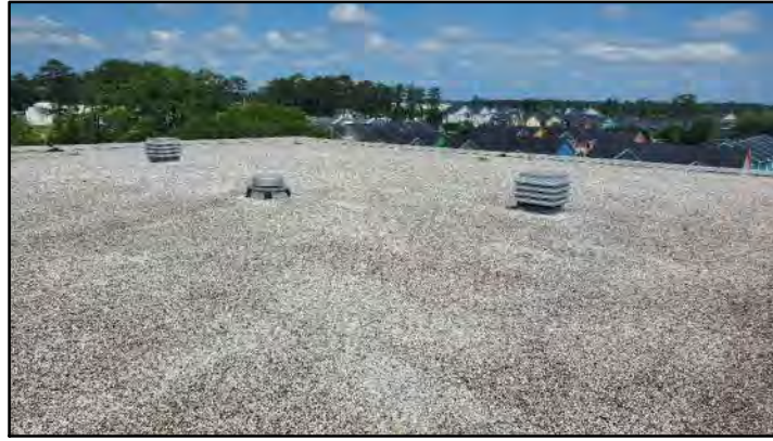
PHOTO # 14 ROOF AREA C
