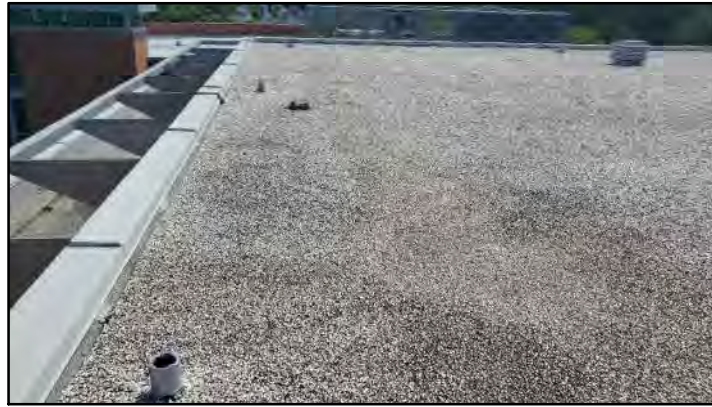
PHOTO # 17 ROOF AREA C
