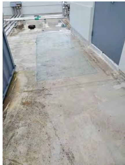
PHOTO # 10 ROOF AREA G
