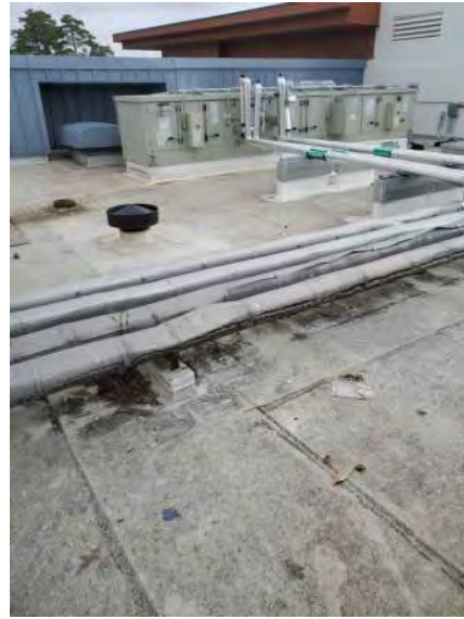
PHOTO # 3 ROOF AREA F
