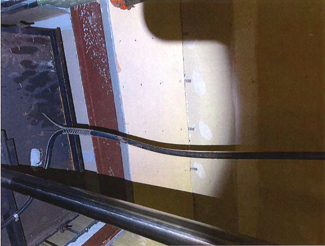
Picture of elevator shaft
