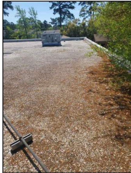
PHOTO # 5 ROOF AREA D
