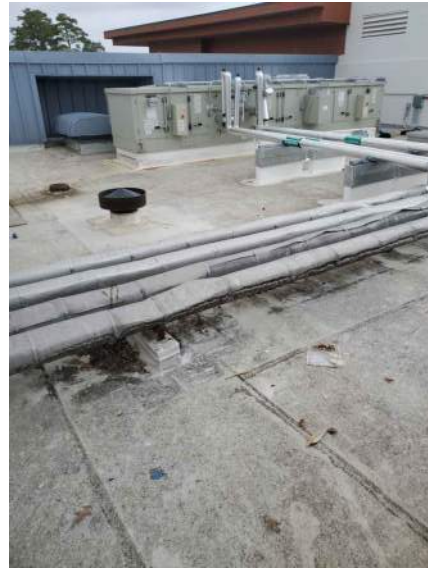
PHOTO #3 ROOF AREA F
