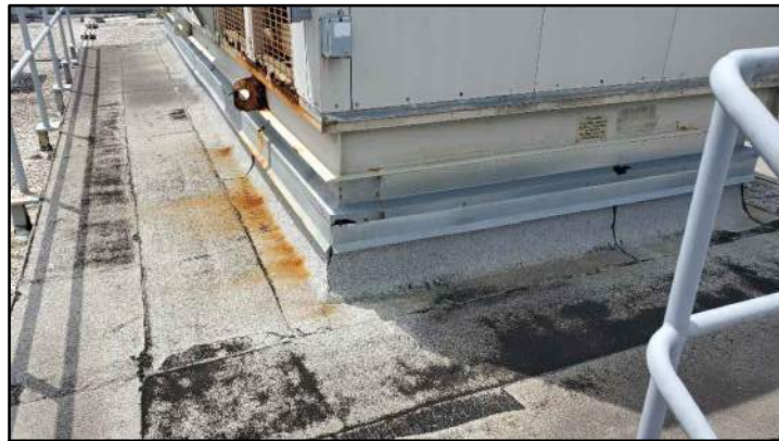
PHOTO # 11 ROOF AREA B1
