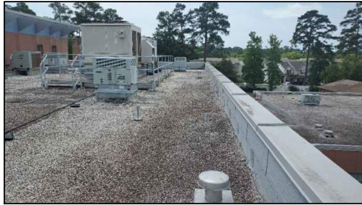
PHOTO # 5 ROOF AREA B
