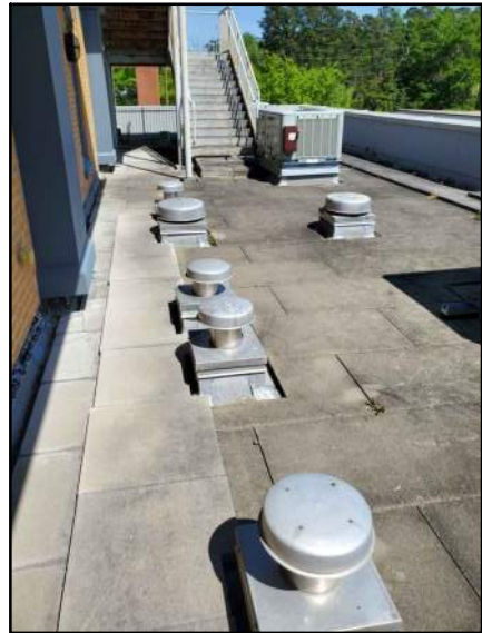
PHOTO # 5 ROOF AREA E
