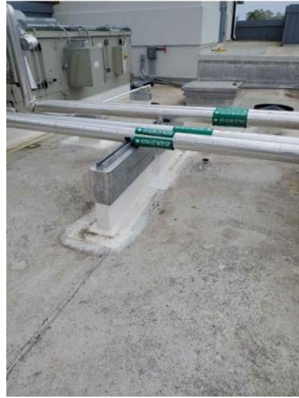
PHOTO #7 ROOF AREA F
