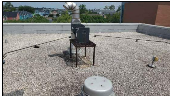
PHOTO # 9 ROOF AREA B
