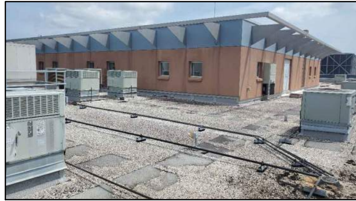
PHOTO # 6 ROOF AREA B
