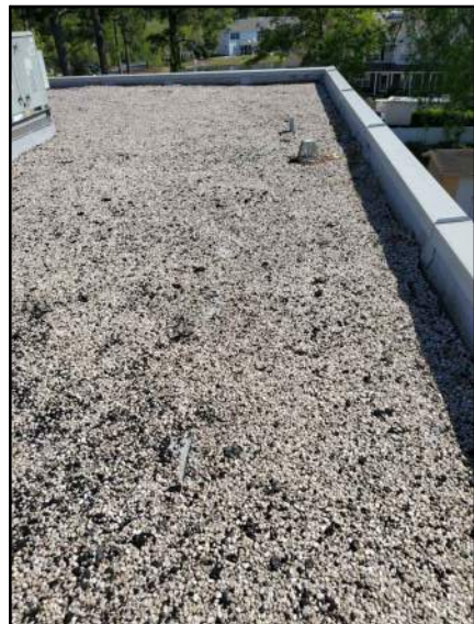
PHOTO # 22 ROOF AREA F
