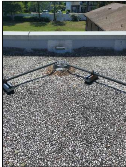
PHOTO # 6 ROOF AREA D
