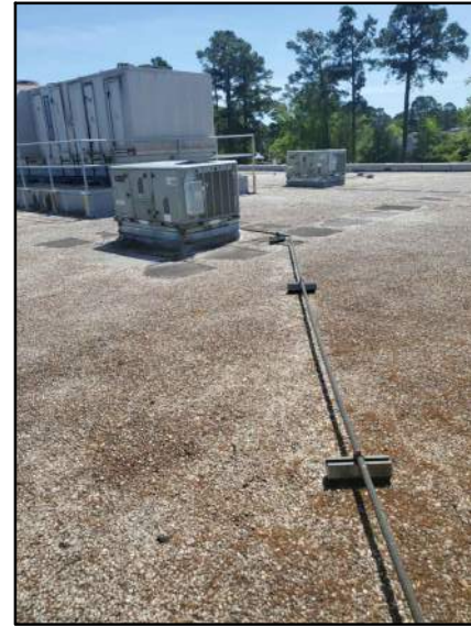
PHOTO # 4 ROOF AREA D
