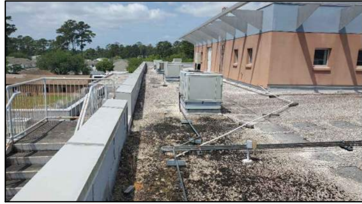
PHOTO # 1 ROOF AREA B
