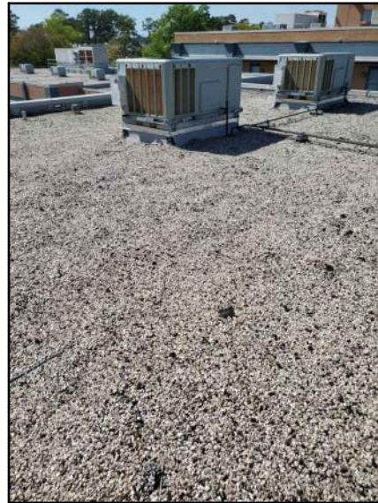
PHOTO # 19 ROOF AREA F
