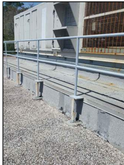
PHOTO # 11 ROOF AREA D2
