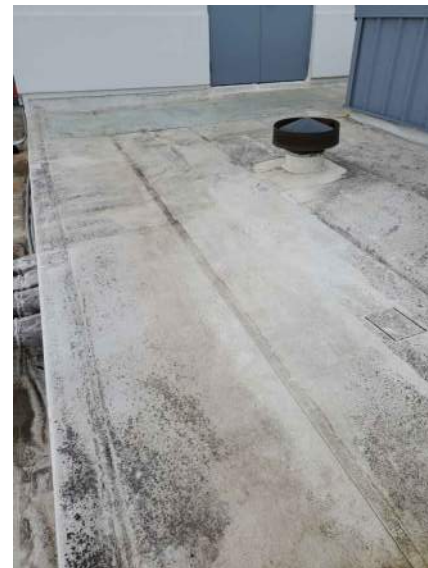
PHOTO #12 ROOF AREA G
