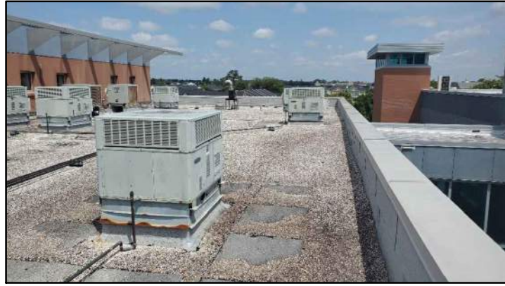
PHOTO # 2 ROOF AREA B
