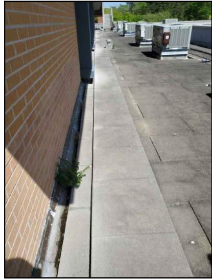
PHOTO # 1 ROOF AREA E
