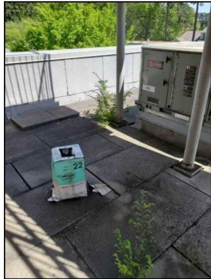
PHOTO # 6 ROOF AREA E
