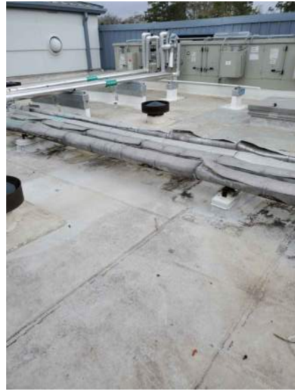
PHOTO #1 ROOF AREA F
