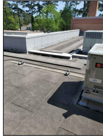
PHOTO # 4 ROOF AREA E
