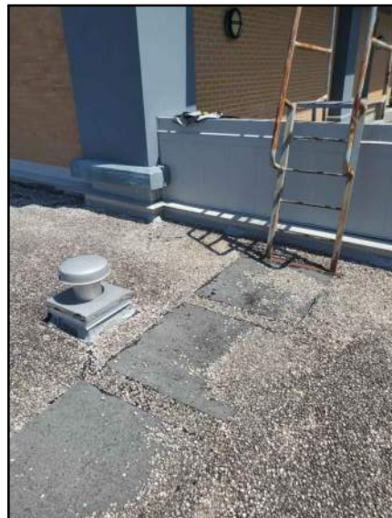
PHOTO # 9 ROOF AREA D1
