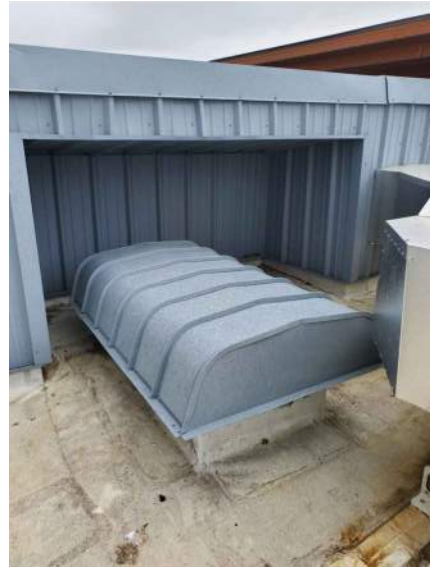
PHOTO #5 ROOF AREA F
