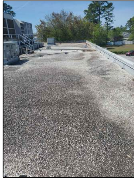
PHOTO # 3 ROOF AREA D
