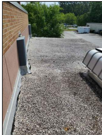
PHOTO # 11 ROOF AREA E2
