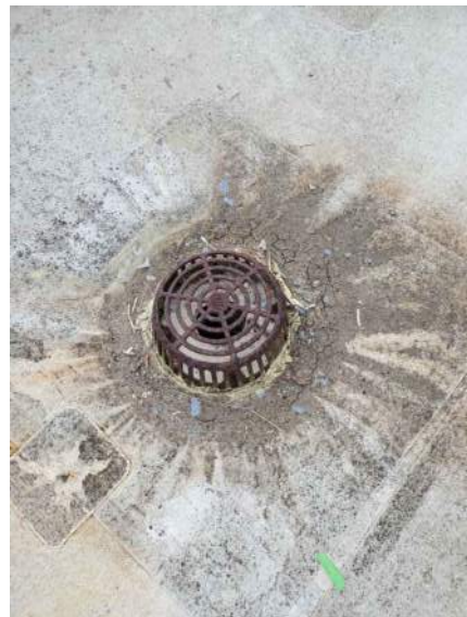
PHOTO #9 ROOF AREA F
