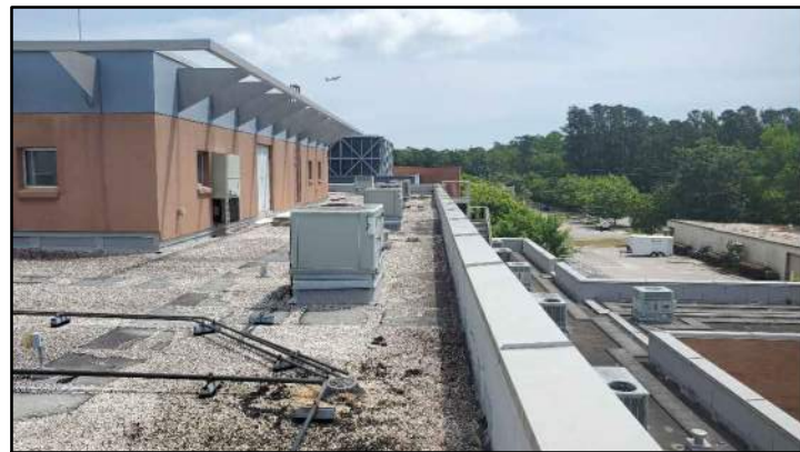
PHOTO # 7 ROOF AREA B
