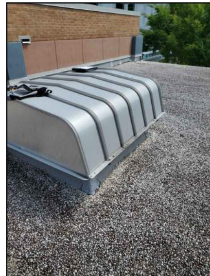
PHOTO # 12 ROOF AREA E2
