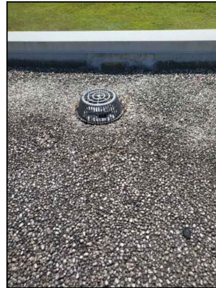
PHOTO # 8 ROOF AREA D1
