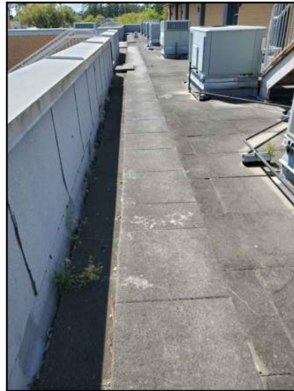
PHOTO # 7 ROOF AREA E
