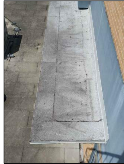
PHOTO # 16 ROOF AREA E4
