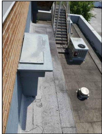
PHOTO # 17 ROOF AREA E4
