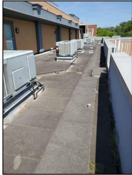
PHOTO # 2 ROOF AREA E
