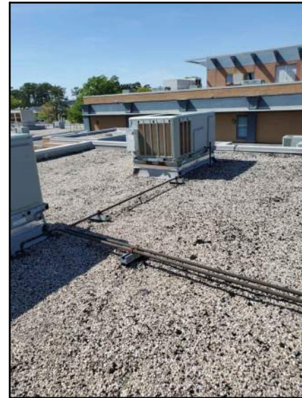
PHOTO # 20 ROOF AREA F
