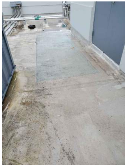
PHOTO #10 ROOF AREA G
