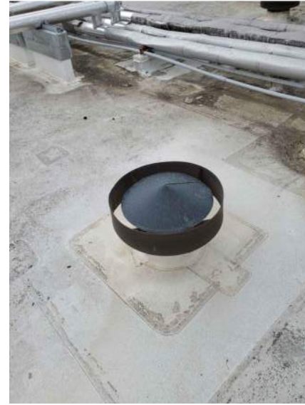
PHOTO #8 ROOF AREA F
