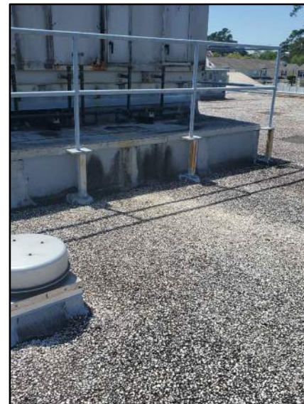
PHOTO # 12 ROOF AREA D2
