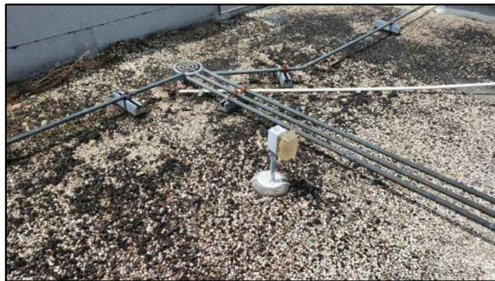
PHOTO # 8 ROOF AREA B
