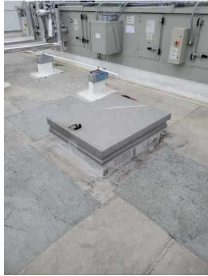
PHOTO #6 ROOF AREA F
