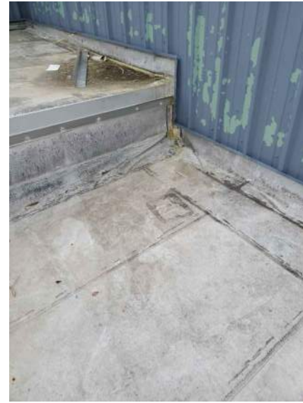
PHOTO #4 ROOF AREA F
