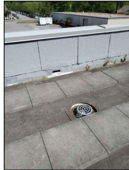
PHOTO # 8 ROOF AREA E
