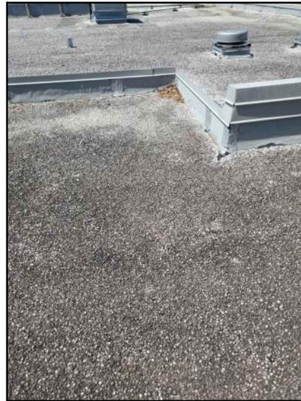
PHOTO # 7 ROOF AREA D1
