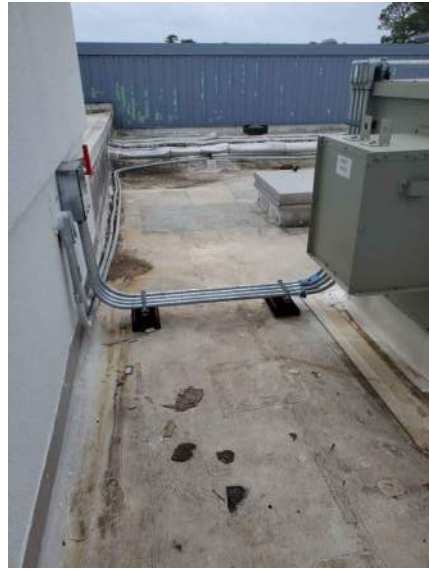
PHOTO #2 ROOF AREA F
