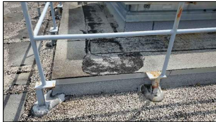
PHOTO # 12 ROOF AREA B1
