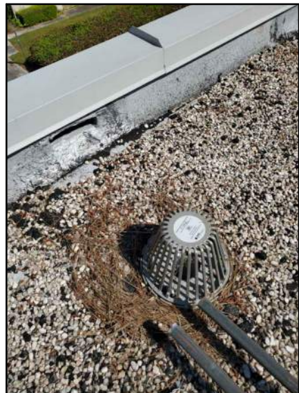
PHOTO # 21 ROOF AREA F
