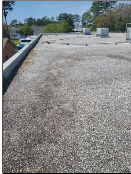
PHOTO # 1 ROOF AREA D
