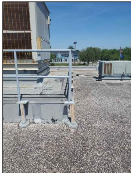
PHOTO # 10 ROOF AREA D2
