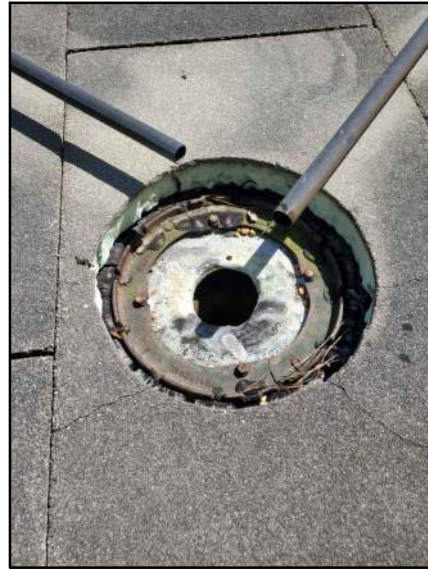
PHOTO # 3 ROOF AREA E
