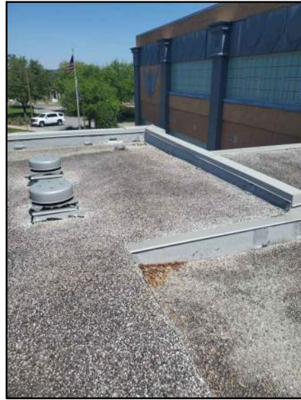
PHOTO # 2 ROOF AREA D
