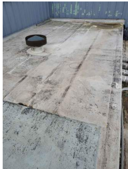
PHOTO #11 ROOF AREA G
