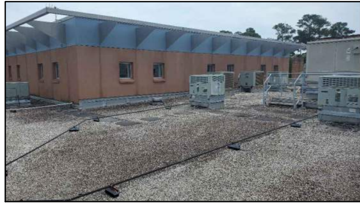
PHOTO # 4 ROOF AREA B
