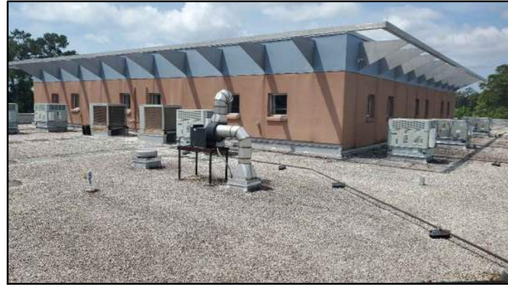
PHOTO # 3 ROOF AREA B
